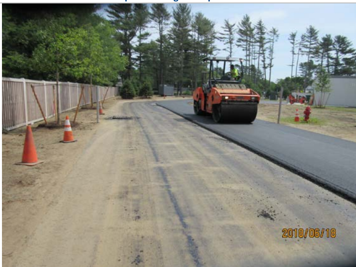
Asphalt Paving at Loop Road
