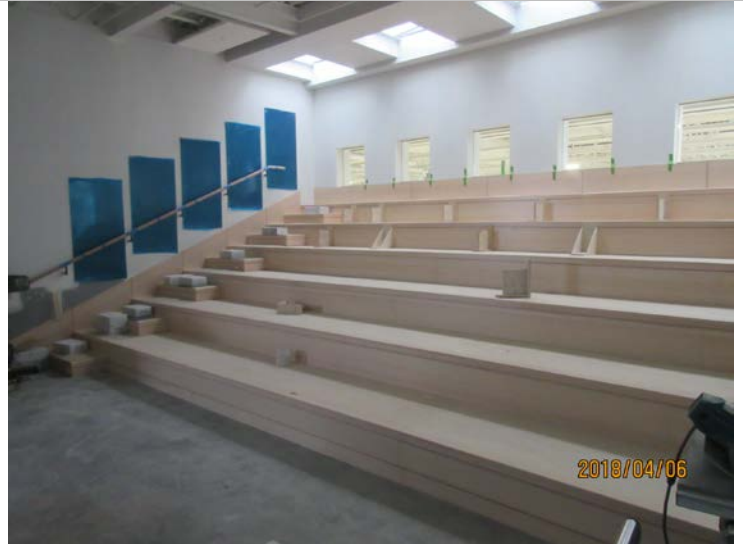
Millwork Installation at Proscenium
