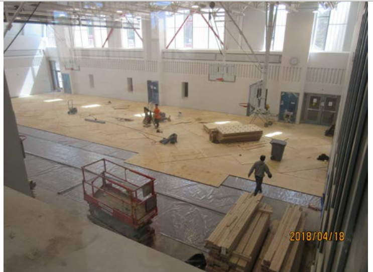
Sub-Floor Installation at Gymnasium
