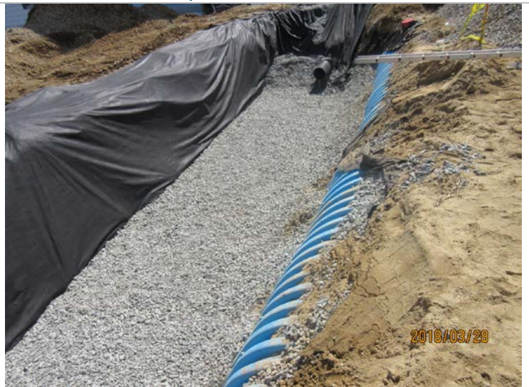
Cultec System Installation and Backfill
