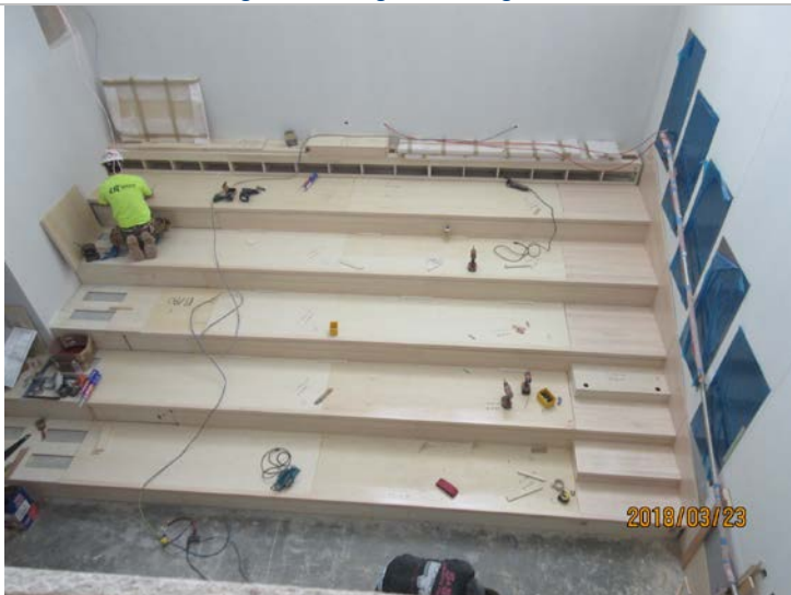
Gathering Area Framing and Flooring Installation
