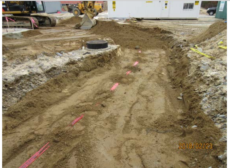
Irrigation Main Backfill at Pre-K
