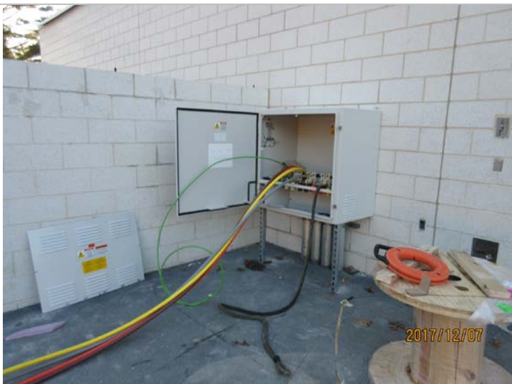
ELETRICAL FEED PULL FROM GENERATOR
