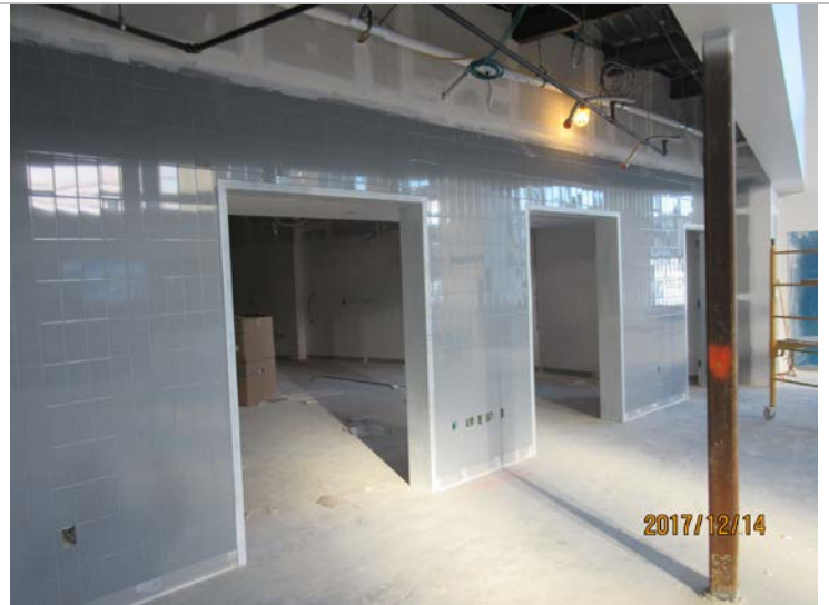
TYPICAL CLASSROOM MARKERBOARD/MILLWORK & FLOOR PREP
