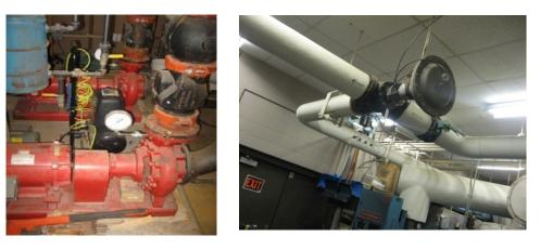
off the header is maintained by a cross over valve located in the mechanical room near the pumps (see Picture). The motors are old and not energy efficient.
