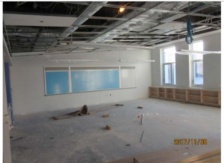
MARKERBOARD INSTALLATION IN TYPICAL CLASSROOM
