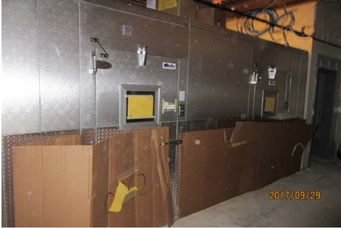
Walk-In Cooler & Freezer Installation
