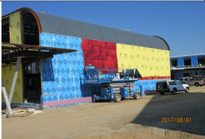
Air Vapor Barrier at Gymnasium Wall
