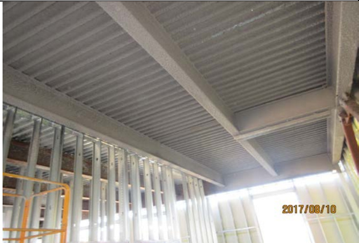
Spray On Fire Proofing Application
