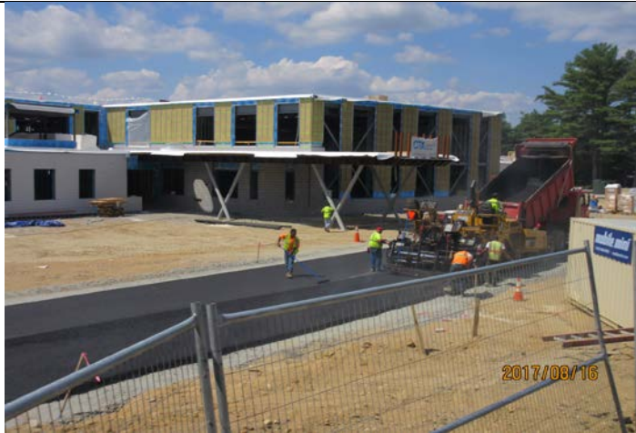
Asphalt Binder Course Installation
