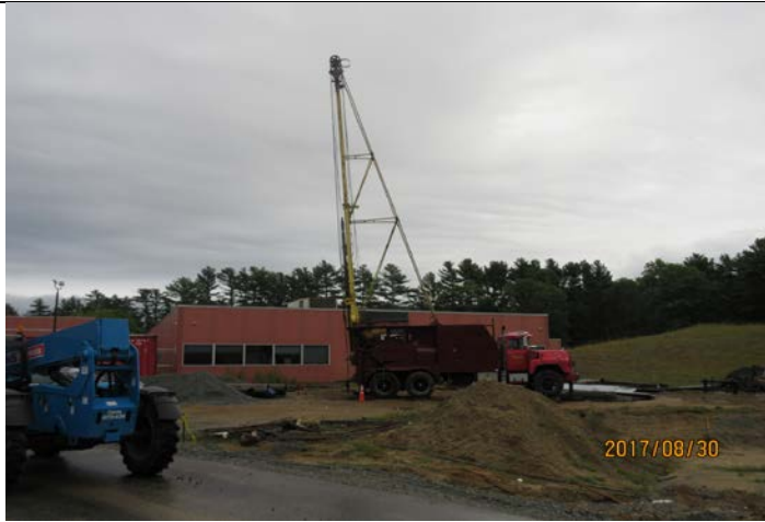
Installation of Irrigation Well
