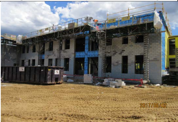
Air Vapor Barrier & Masonry installation at 'B' Wing
