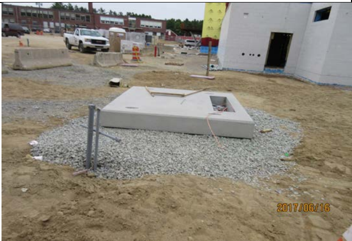
Generator Pad Installation
