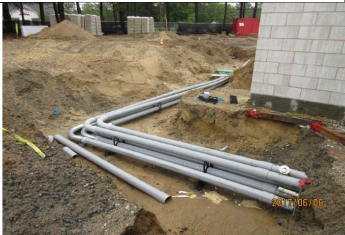
Electrical Duct Bank Installation at Northeast Elevation
