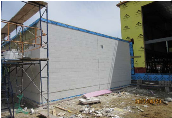
Masonry Block Installation at 'A' Wing North Elevation
