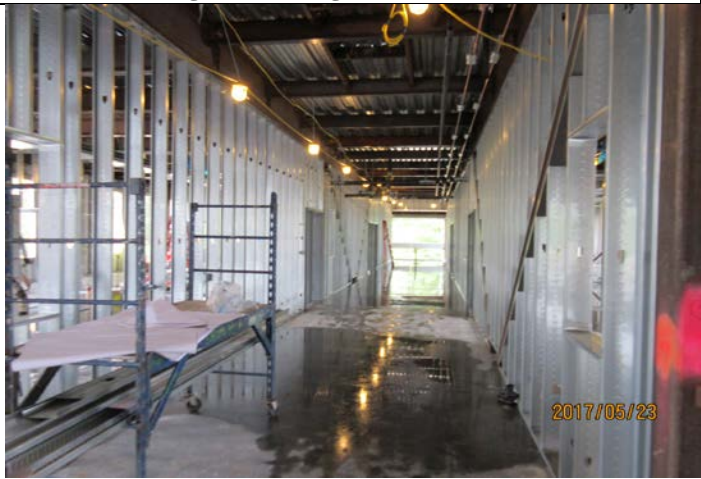
Interior Framing at 'A' Wing Corridor
