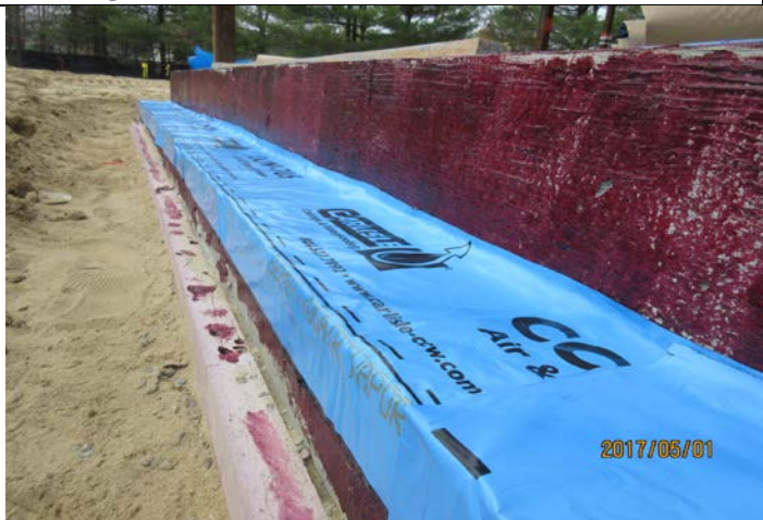
'A' Wing Brick Shelf AVB Installation
