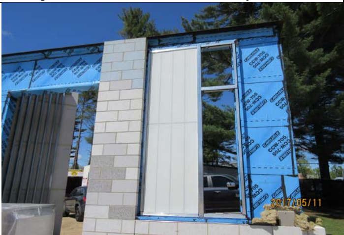
Mockup Installation of Translucent Panel System
