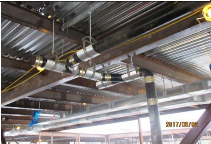
Rain Leader Piping Installation at 2 nd Floor 'A' Wing
