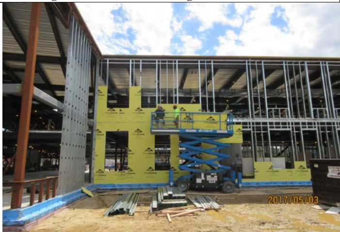
Sheathing Installation at 'A' Wing North Elevation
