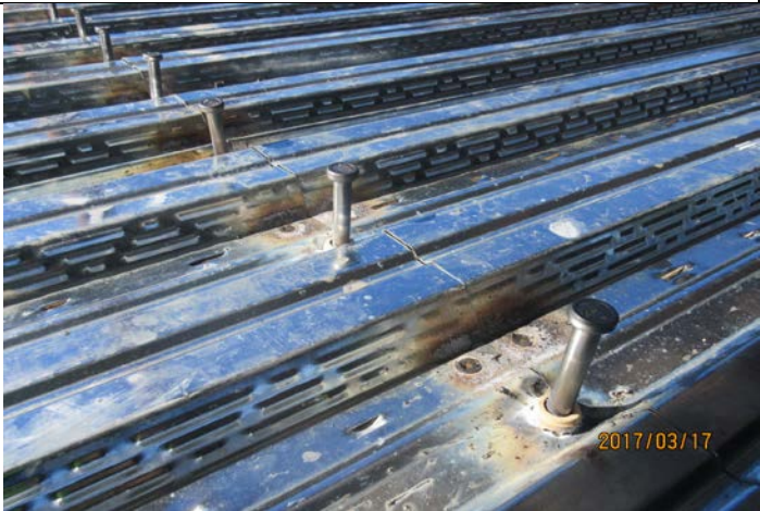
Shear Stud Welding for Decking at A Building
