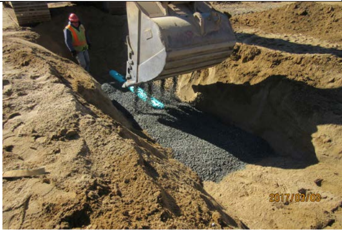
Backfill Site Drainage at East Elevation
