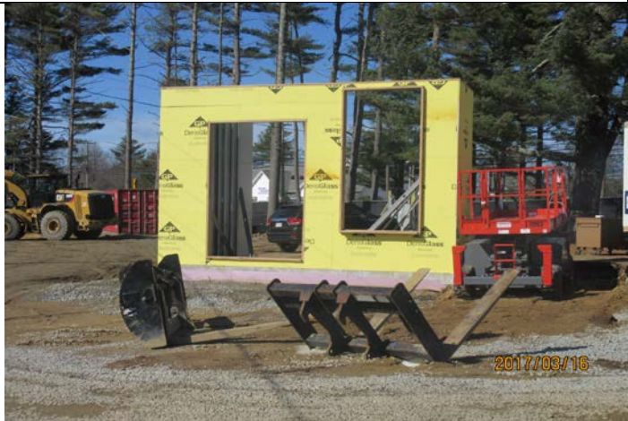
Exterior Sheathing & Window Framing at Mockup
