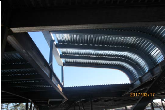
Rolled Deck at Gymnasium Roof
