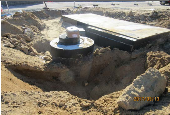
Sanitary and Waste Underground Tanks Installed
