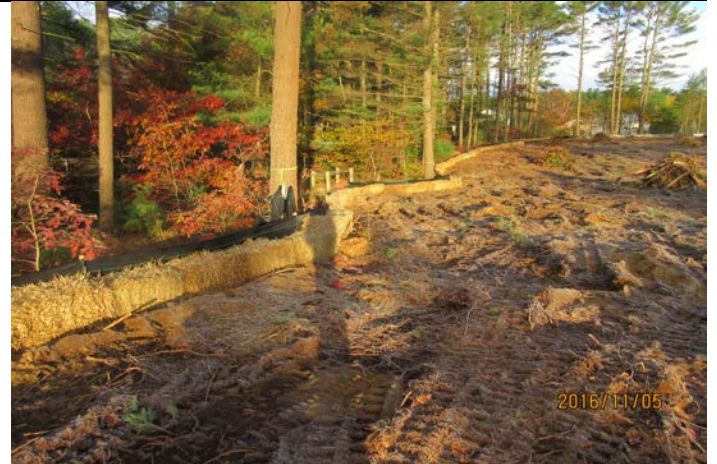
Erosion Controls at Site Perimeter
