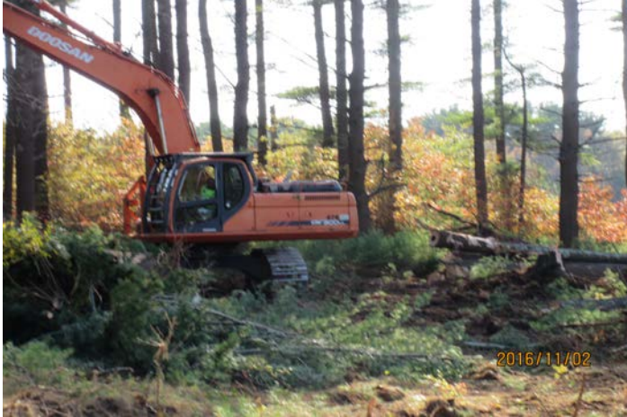
Phase I Tree Clearing at Southwest
