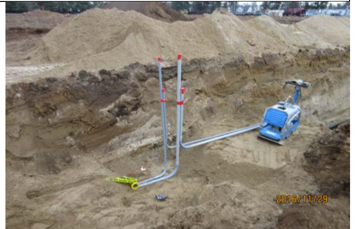
Power and new Water Line Backfill & Compaction
