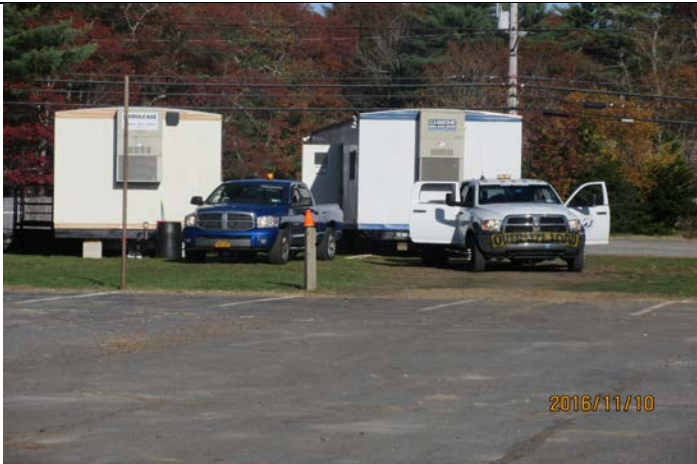
Construction Trailers Delivered to Site
