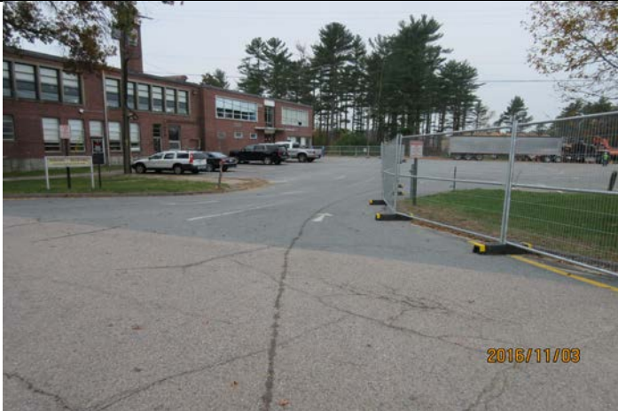
Construction Site Fencing
