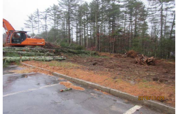
Phase II Tree Clearing at Teacher Parking
