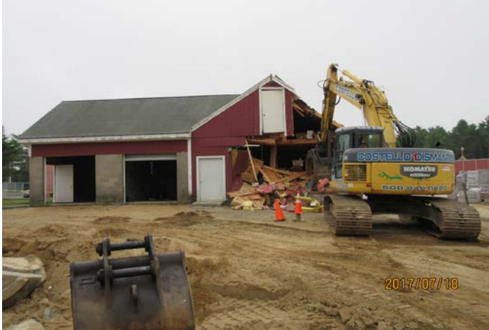
Demolition of Existing Shed
