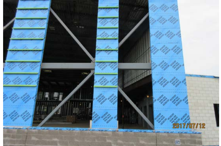
Air Vapor Barrier & Green Girt Installation at Cafeteria
