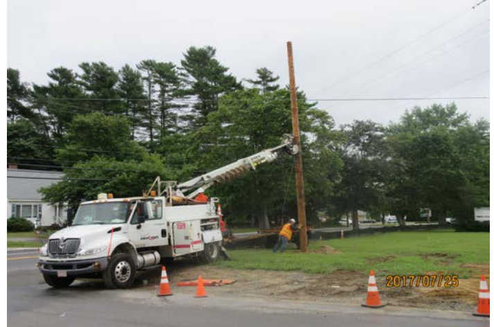
Tel/Com Utility Pole Installation at Rt. 58
