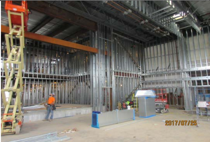
Cafeteria and Multipurpose Room Soffit Framing
