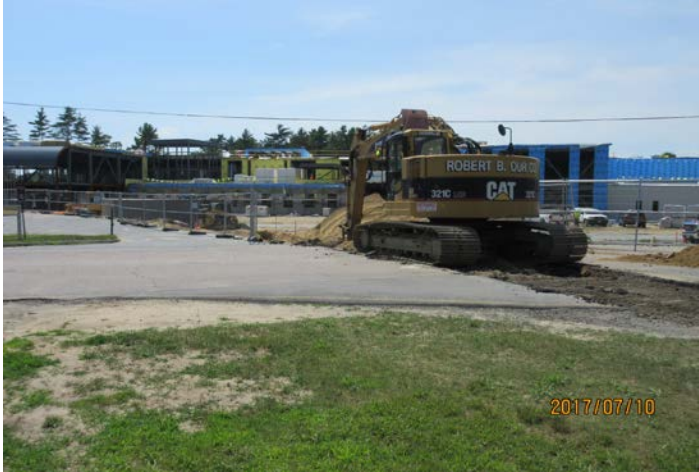
Excavating Trench for New Tel/Com Utility
