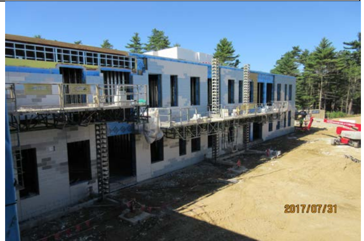
Exterior Masonry/Air Vapor Barrier/Window Install
