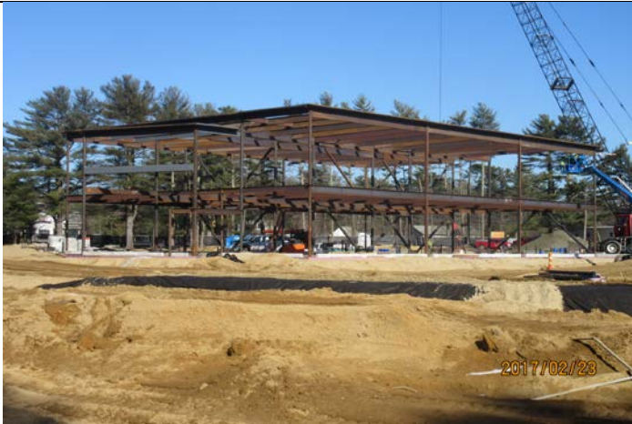
'A' Building Steel Erection Classroom Area
