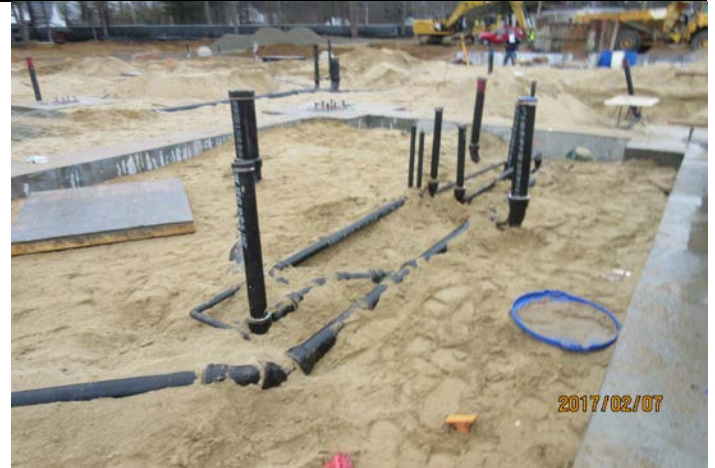
Sanitary and Waste Underground at 'A' Building
