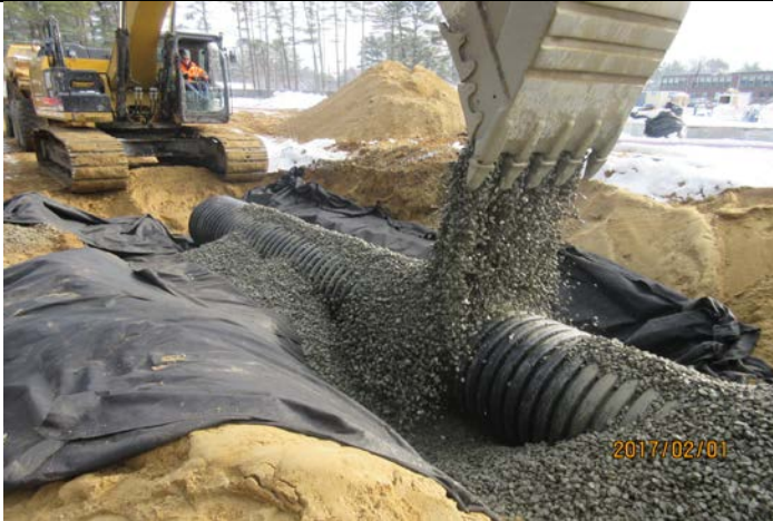
Backfill Site Drainage at West Elevation
