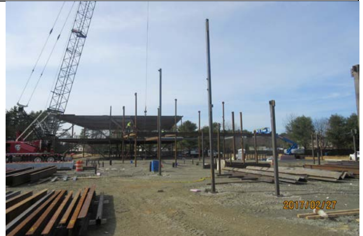
'A' Building Column Erection Near Cafeteria
