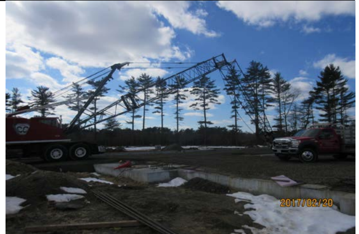
Crane Mobilization and Setup
