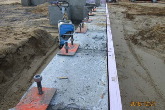
Anchor Bolt Plates & Soil Compaction at Foundation
