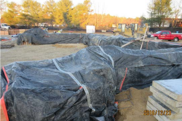
Cold Weather Concrete Protection at Foundations
