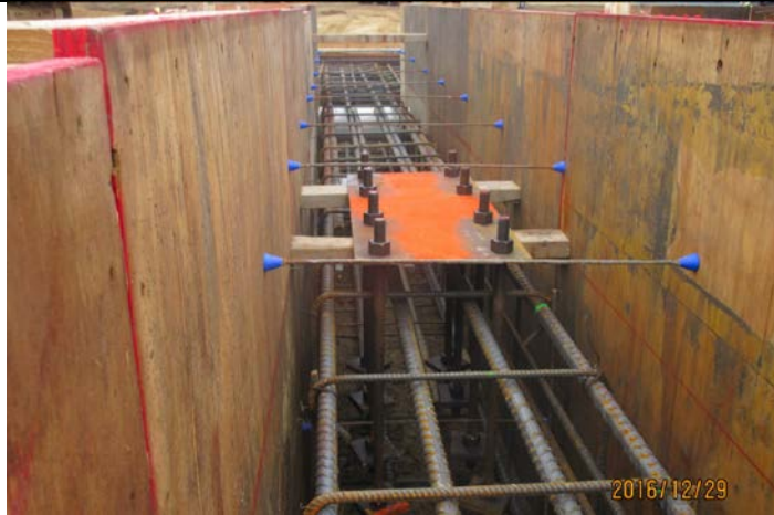
Rebar Inspection at Column Base Plate
