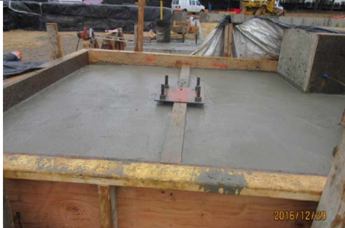
Column Baseplate Concrete Footing
