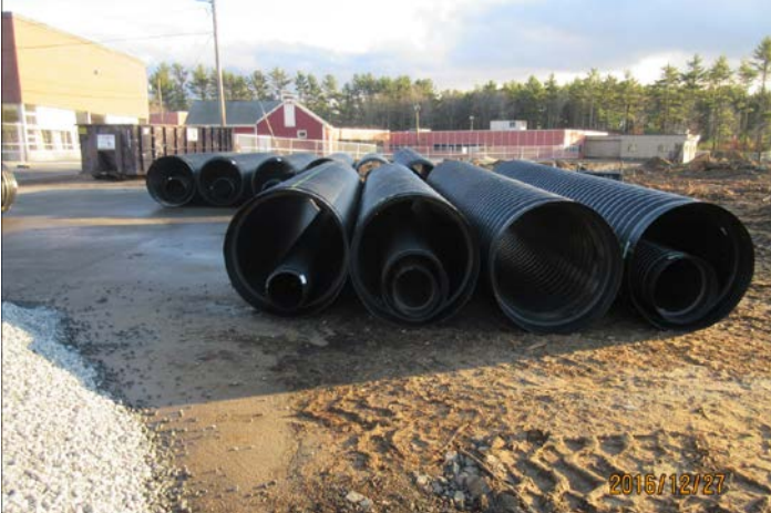
Subsurface Infiltration Materials
